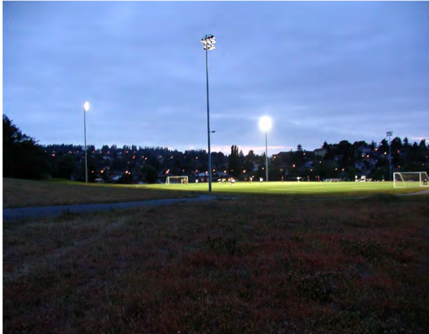
Urban soccer field with 4th generation spill and glare control fixtures illuminated to 200 lux. Photo taken approximately 50 metres from the edge of the field.
